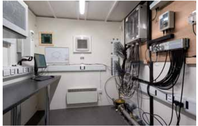
Inside one of the remote monitoring stations
