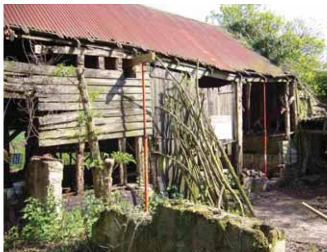
Orchard Barn pre-restoration
