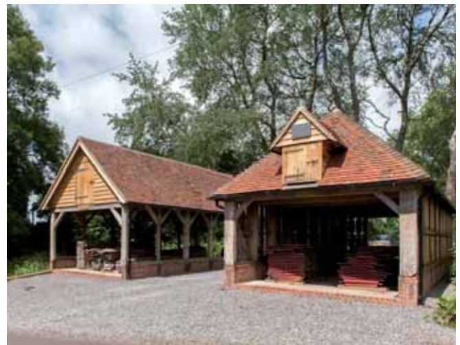
The relocated and restored timber-drying sheds
