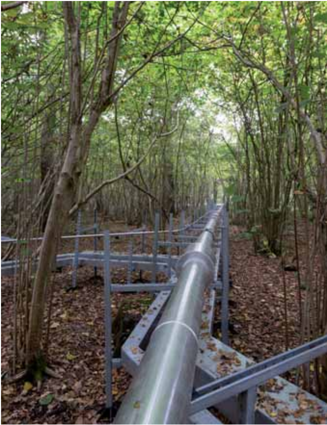
The liquid CO 2 is transported in pipes supported by minimal impact frames
